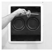
Protect the drivers with the paint mask and remove grille before painting the baffle edge as well as the grille as necessary.
